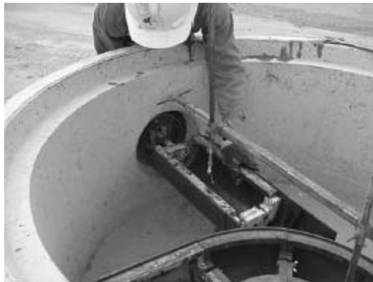
#4 POSITION ANTI FLOTATION BAR AND ADDITIONAL CHANNEL
