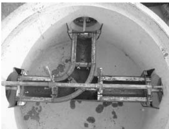
#6 COMPLETED THREE-WAY ASSEMBLY READY TO POUR
