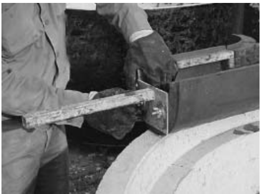
#2 ASSEMBLE SMALLEST ANGLE WITH CENTERING ADAPTOR
